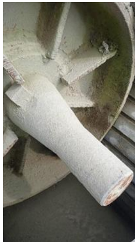
Gambar 1. Kerusakan Drum Pulley.
